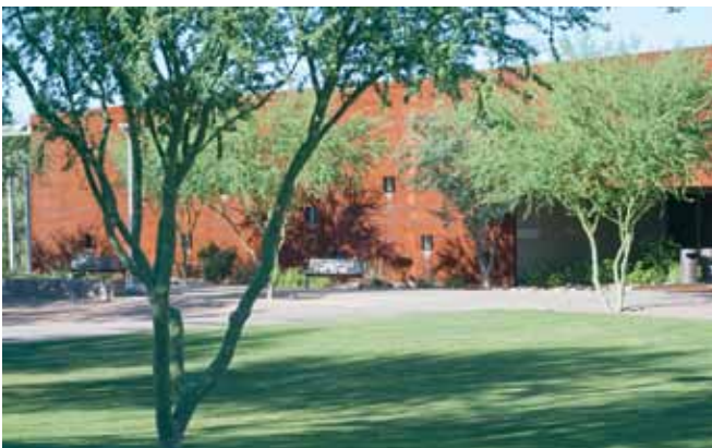
Chinle Student Services Building at GCC North
