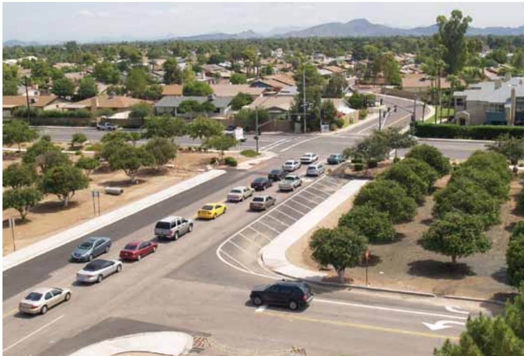
Facing roughly northeast, this is a view of the newly widened entrance to the north parking lot at the intersection of 59th Avenue and Vogel
